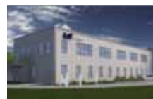
LS EV Poland./LSCP (Dzierzoniow) Automotive battery components Optical cable
