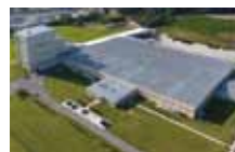
LSCUS(Tarboro) MV / LV cable Control, Instrument cable
