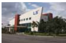
LSCV(HO Chi Minh) MV / LV cable UTP, Optical cable Overhead cable
